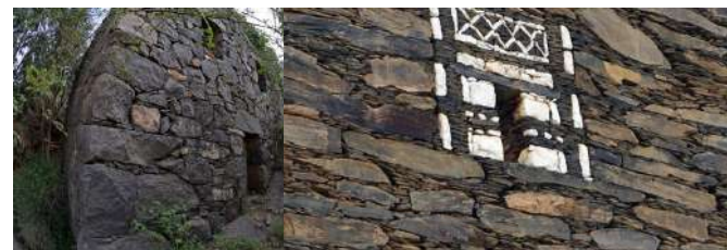
Rock Building sttrcuture
